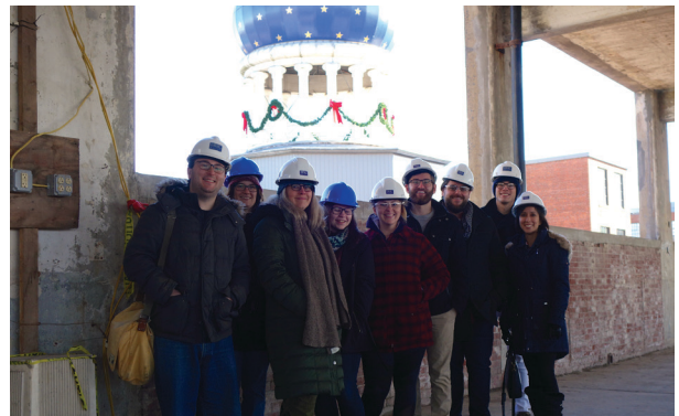
My fall 2018 Historic Preservation Law class at the construction site for the North Army of Colt Gateway project, one of the most significant historic preservation rehabilitations in the state. Each of my students picked a Hartford historic site and wrote a paper on it; one of the students wrote about the application of historic tax credit law to the first phases of the Colt rehabilitation.
